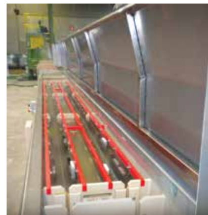
Zinc on Steel + OTO H2
